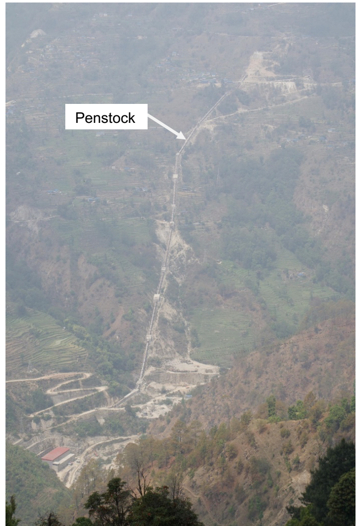
Figure 1. Penstock Alignment.
