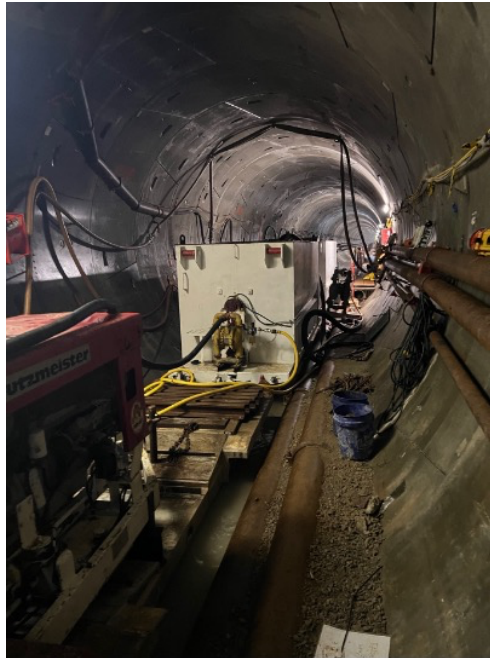
Figure 1. Grouting operations at Adit 9.
