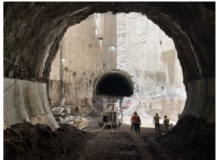
Figure 2. Bench excavation of Tail Tunnel viewed from Starter Tunnel.
