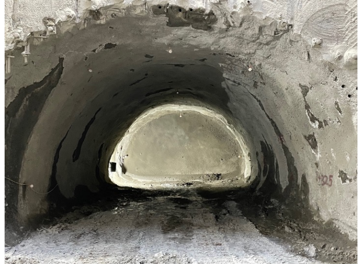
Figure 1. Completed Tail Tunnel top heading.
