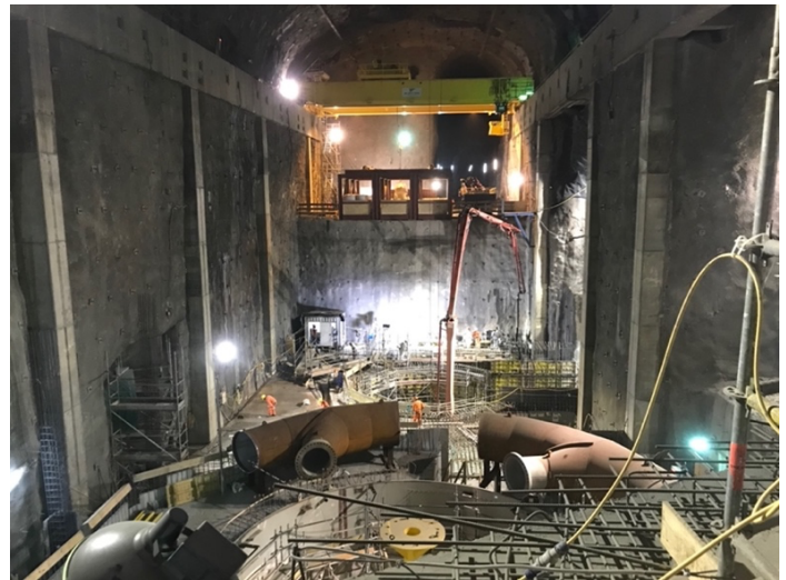
Figure 1. Powerhouse Las Lajas Cavern.
