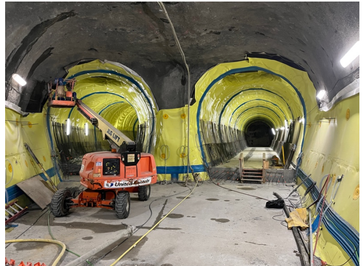
Figure 2. Installation of waterproofing in Bifurcation.
