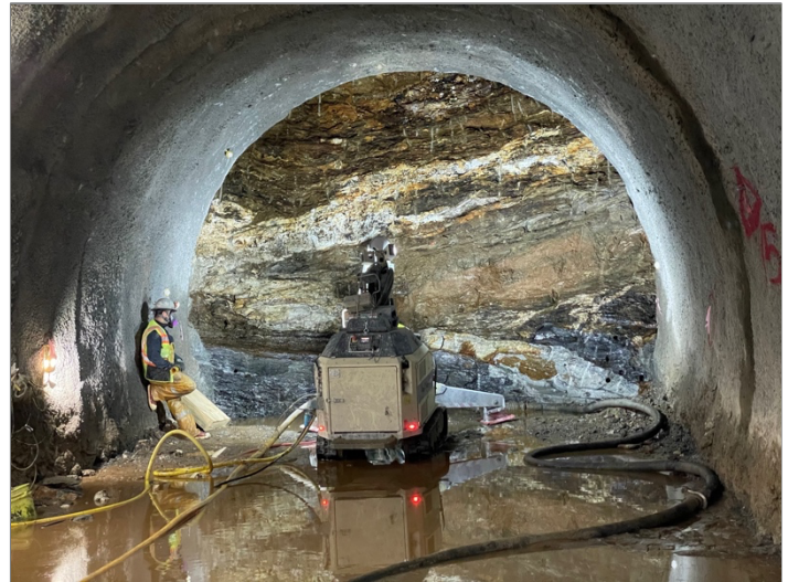
Figure 1. Weathered Gneiss exposed at excavation face.
