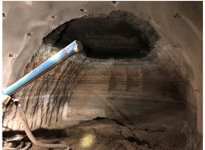
Figure 2. West tunnel face.
