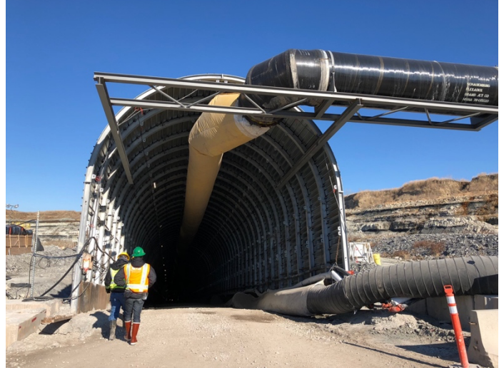
Figure 1. East tunnel portal.
