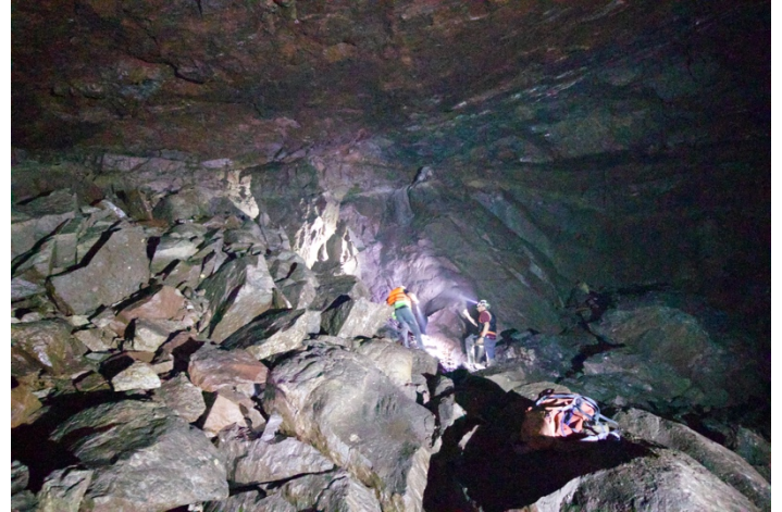
Figure 1. Resulting Cavern from tunnel collapse.
