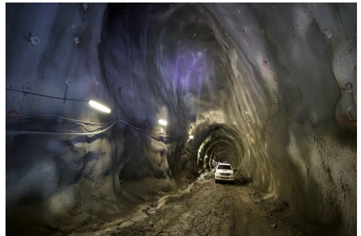
Figure 2. Repaired section of major rock fall.
