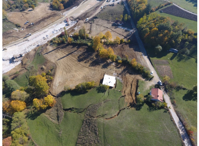
Figure 1. Drone picture showing landslide (courtesy BEGP).
