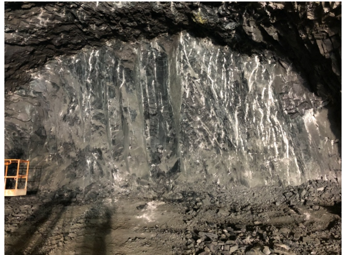
Figure 2. Top heading excavation face.
