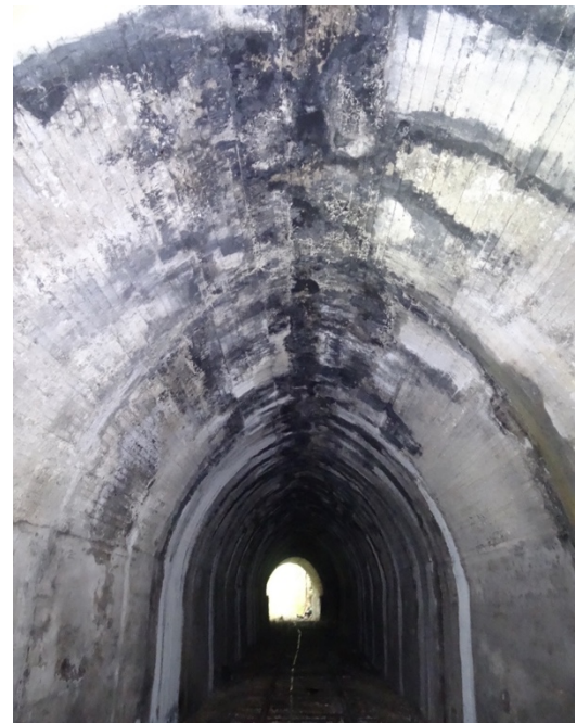
Figure 2. Lined Ramble Tunnel.
