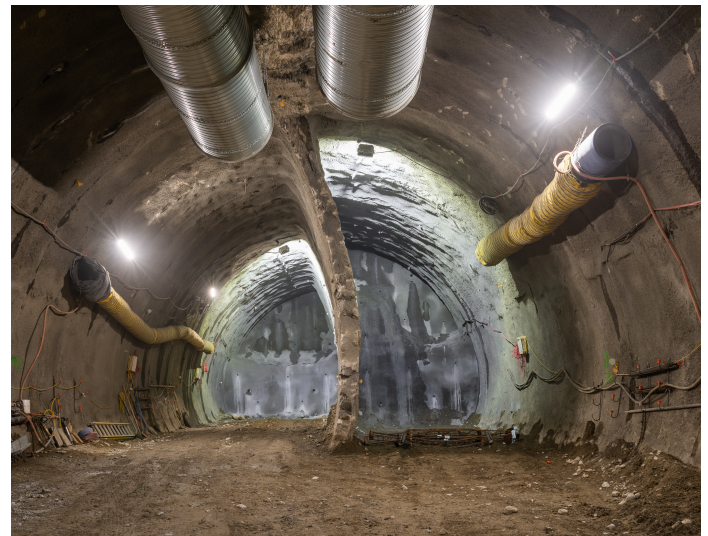
Figure 2. Excavation drifts of SEM portion of Downtown Bellevue Tunnel.
