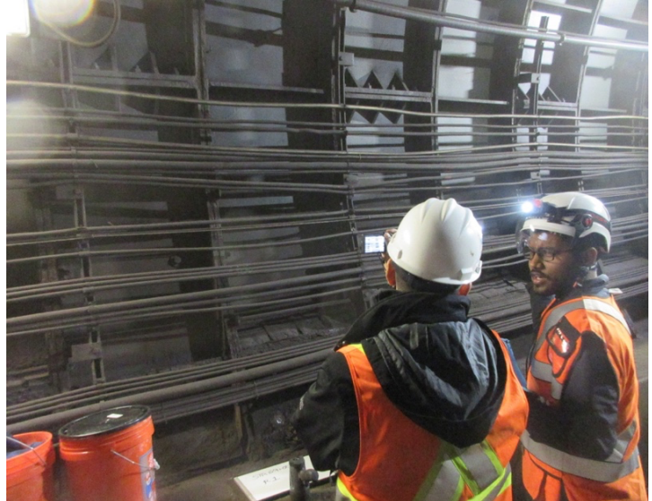
Figure 1. GZ inspector evaluating condition of steel tunnel liner.
