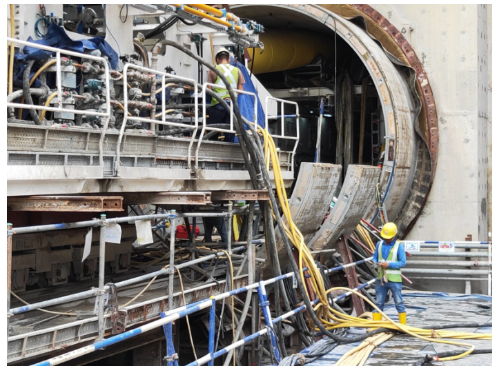
Figure 2. TBM Conversion for Woodlands Bound Main Drive (Courtesy of MCC).
