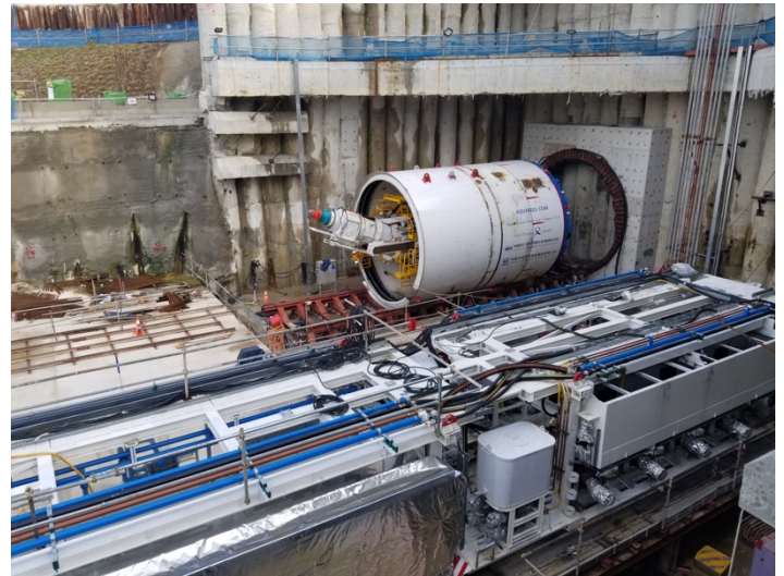
Figure 1. TBM Assembly for Changi Bound Drive (Courtesy of MCC).
