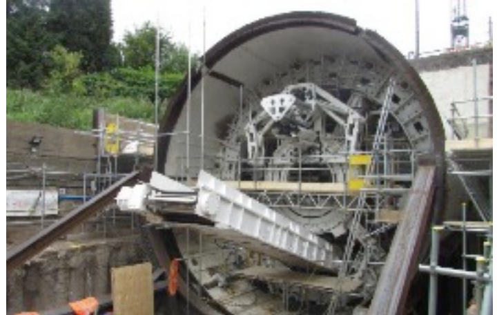
Figure 1. TBM assembly (courtesy OTB Engineering).
