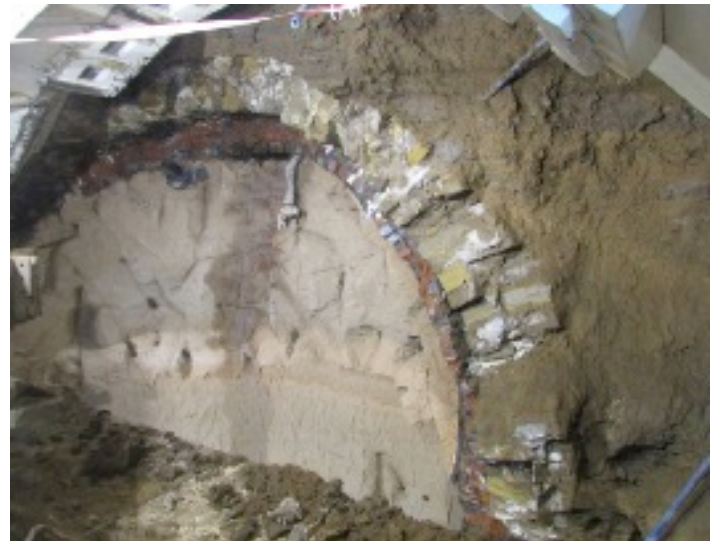
Figure 2. Demolition and enlargement of brick-lined tunnel (courtesy OTB Engineering).
