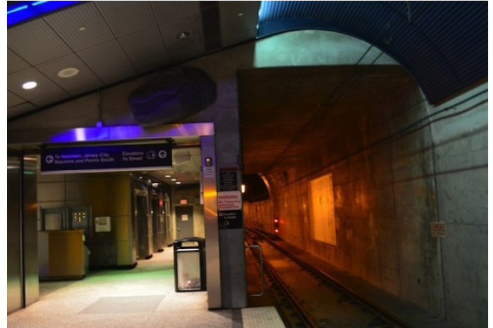
Figure 1. Bergenline Avenue Platform looking west.
