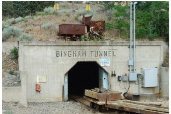
Figure 2. Portal of Bingham Tunnel.
