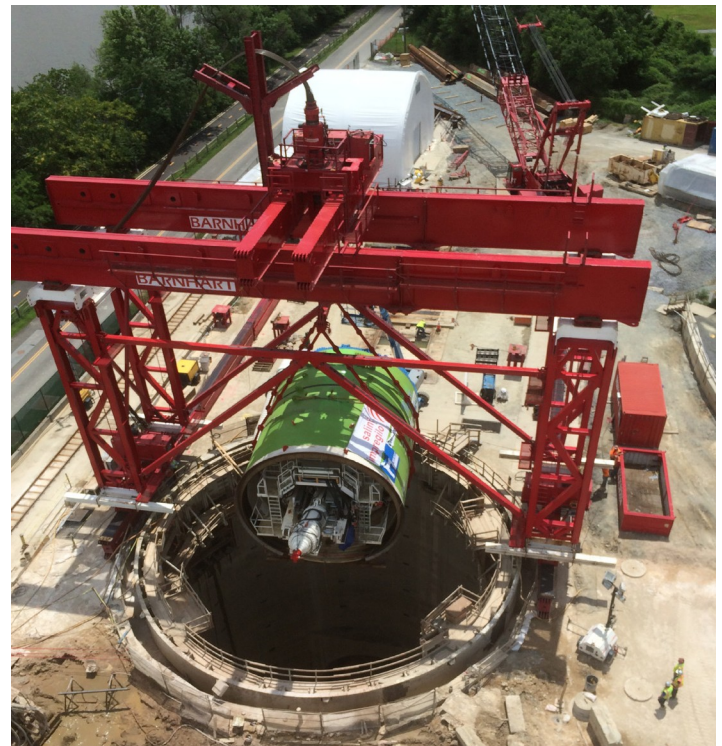
Figure 2. Lowering TBM into the shaft at CSO 019N-DS.
