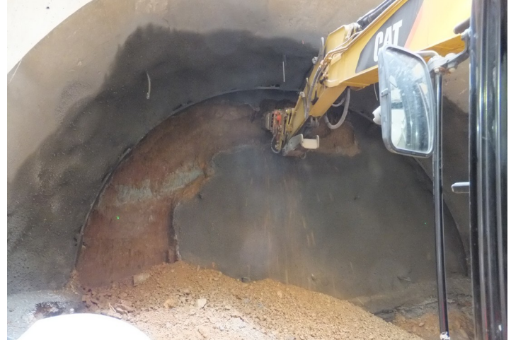
Figure 1. Anacostia River ISCT Excavation.
