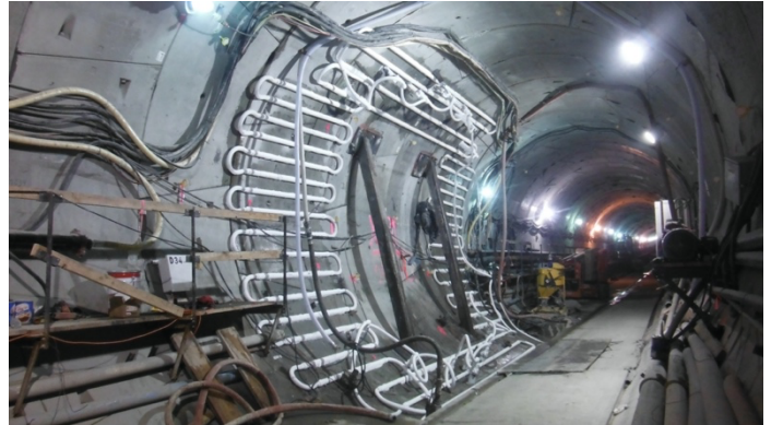
Figure 1. Ground freeze pipe during the ground treatment for the cross passage.
