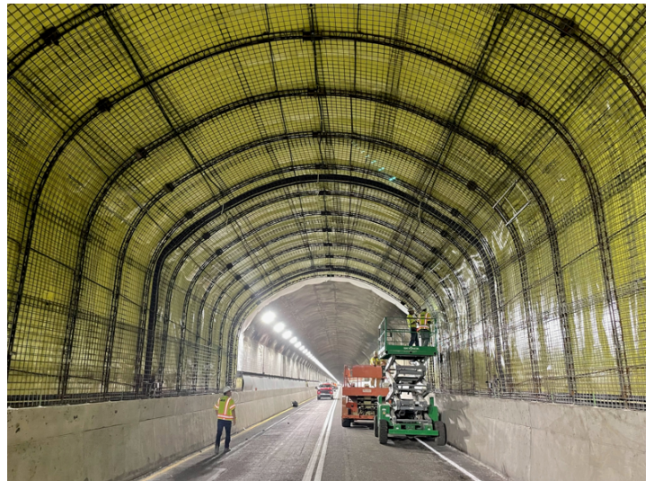
Figure 2. Installed lattice girders and rebar mesh.
