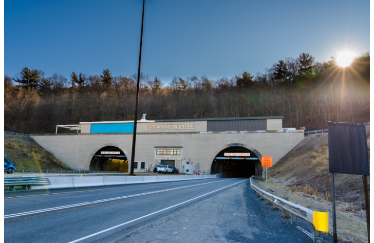
Figure 1. Tuscarora Tunnel Portal
