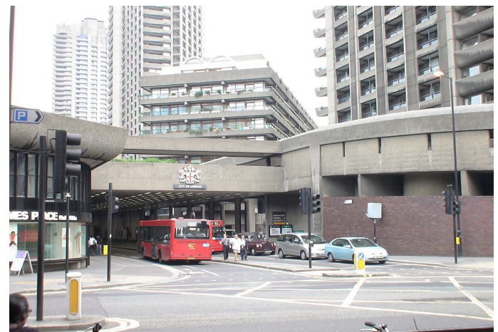
Figure 3. High-rise building along tunnel alignment.
