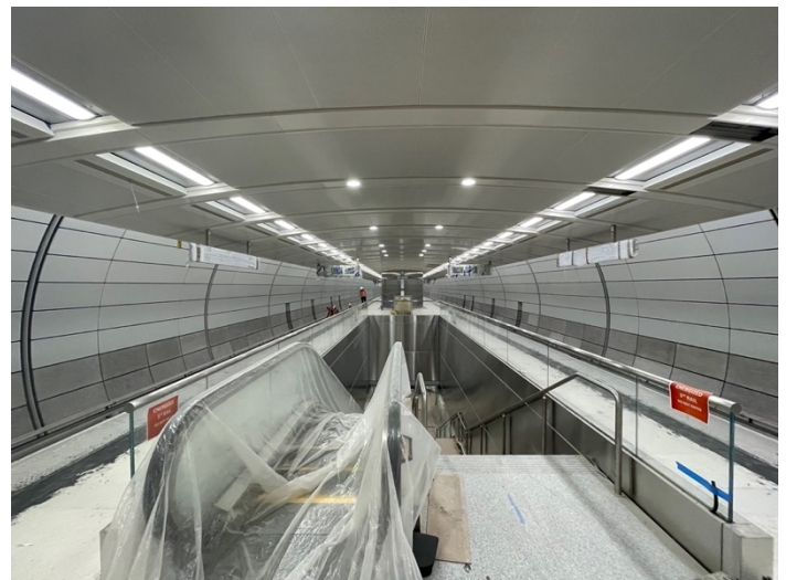
Figure 2. Grand Central Terminal Cavern on Mezzanine level shortly before completion.
