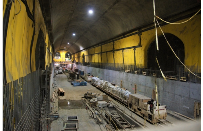
Figure 1. Grand Central Terminal west cavern looking north showing exposed waterproofing.
