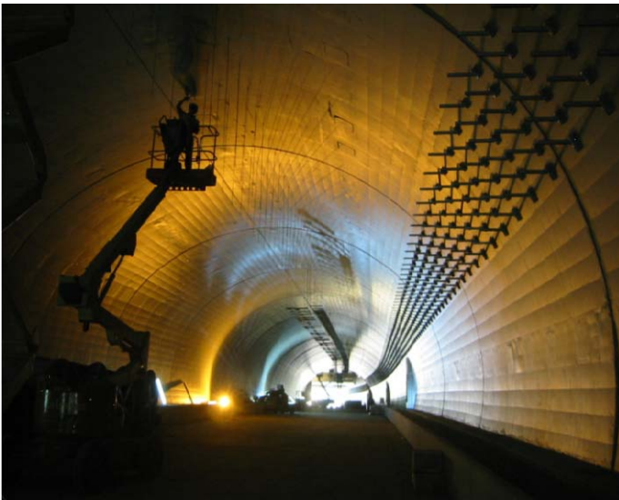
Figure 1: Final Concrete lining and systems installation
