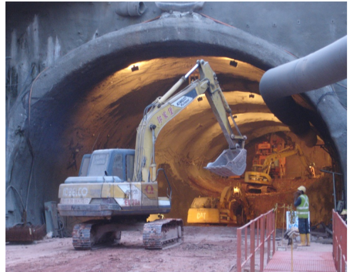
Figure 2: Multiple heading construction under way
